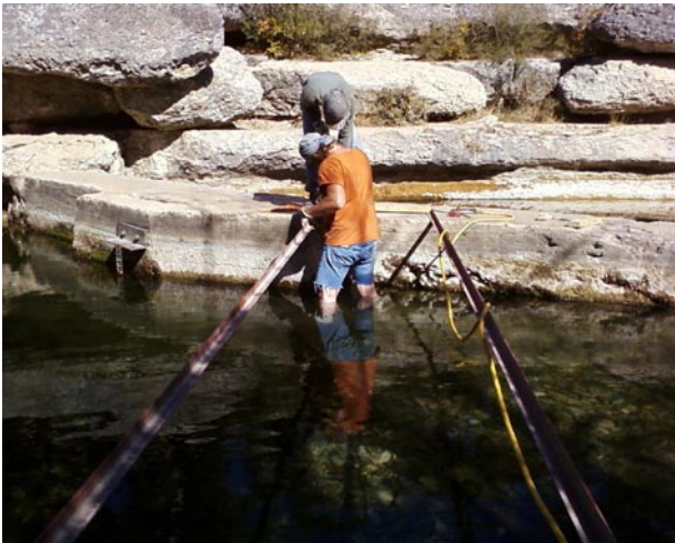
Building the structural support. Photo by Anne Child.
